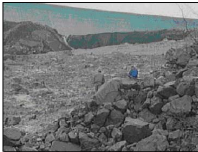
View from inside the emptied reservoir following the 1.5 billion gallon release of water
