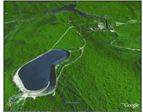
View from above the Taum Sauk upper reservoir
