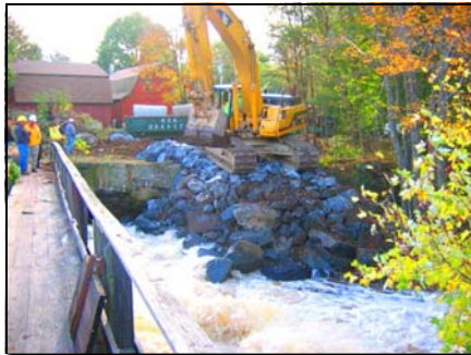
Replacement work gets underway near Taunton, MA after federal EWP funds had been secured.
