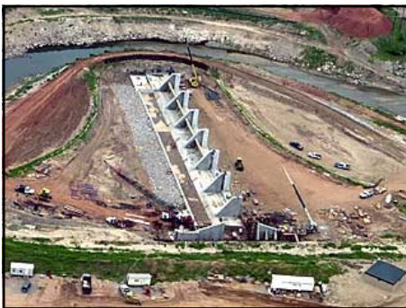
The Oklahoma River was diverted at three locations for construction of low water dams.
